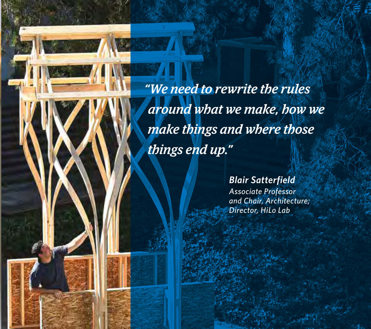
Zippered 2x4s convert waste wood into inspired architecture.
